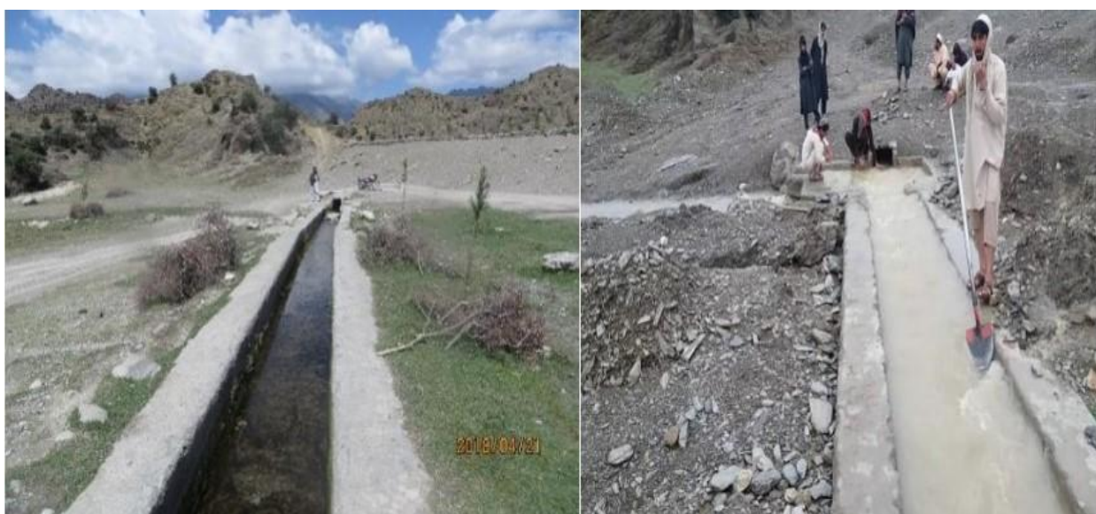
Figure 5. Zambar Karez in Khost Province, discharge before and after rehabilitation (Stanikzai, personal collection, 2020).
