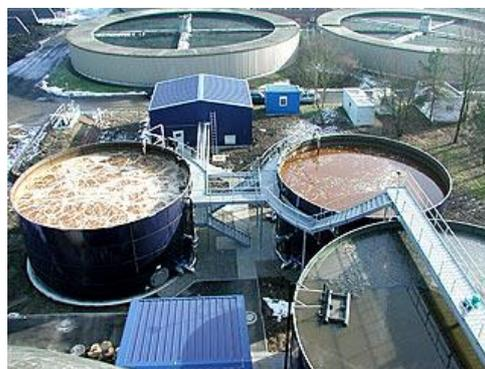
Рисунок 53. – Two SBR Plants for Sludge water Treatment [53]
